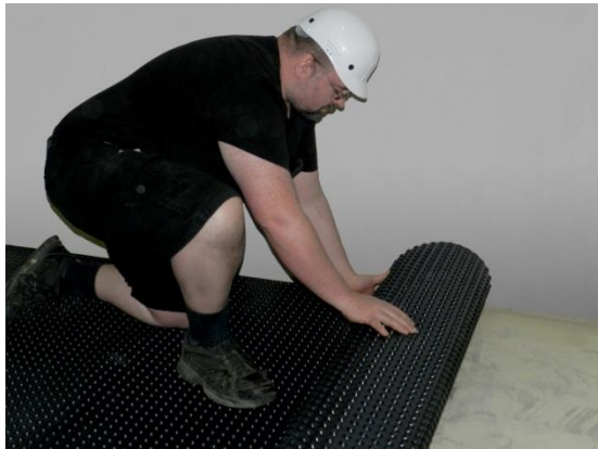
Unroll DMX AG Underlayment™ (dimples facing down).
