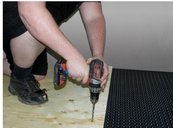
Lay 5/8" plywood or OSB on top of DMX AG Underlayment™. Anchor to the concrete using tap con screws.
